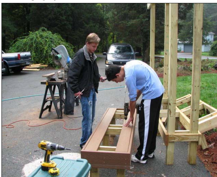
The benches and trellis under construction. Photo by Paula Bramante
