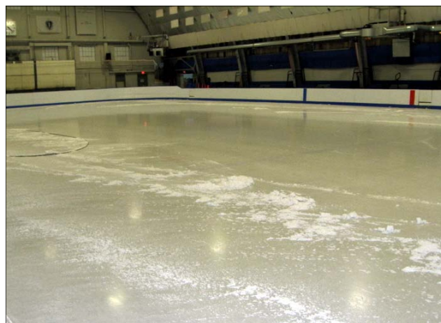
Above, master ice maker Paul Danner edges the ice at 4 am with a special Zamboni tool. Below, the snow left behind after edging. Bottom: the edger leaves a circular, buffed pattern on the ice surface
