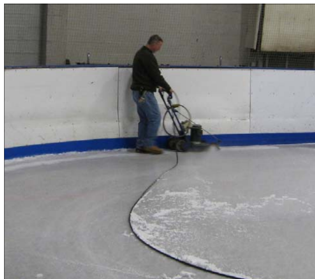
Above, master ice maker Paul Danner edges the ice at 4 am with a special Zamboni tool. Below, the snow left behind after edging. Bottom: the edger leaves a circular, buffed pattern on the ice surface
